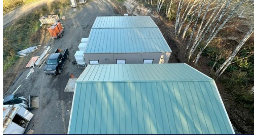
Oregon coast cable landing station
